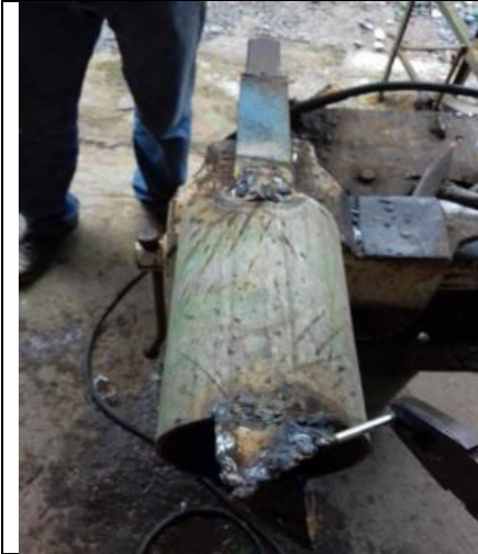
Photo 10. Weld the edge and grind it. Here the cutting tip is a 8 mm concrete drill with a tungsten tip
