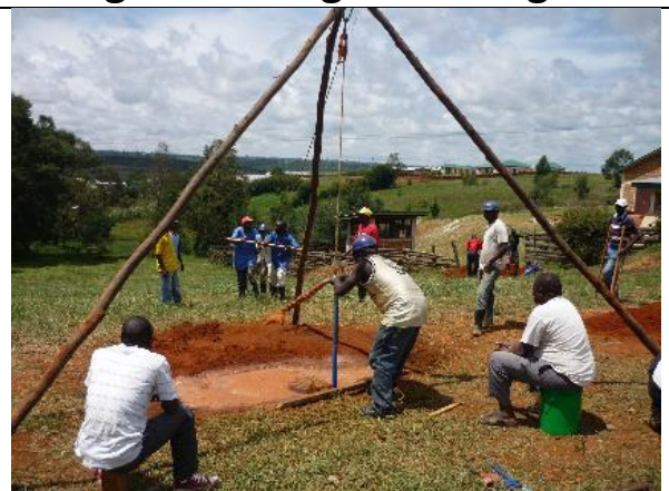
Drilling wells with locally produced tools
