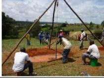
SHIPO manual drilling Ground layers. Hard, no rocks Casings: 1.5- 4 inch Depth: 0-50 m.
