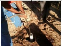
Mzuzu manual drilling Ground layers; Medium hard Casings: 1.5 - 4 inch. Depth: 5- 25 meter Cost/well: \$300 - \$600
