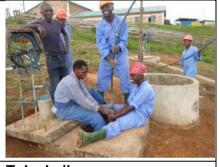
**Tube bailer**Technology to deepen existing wells. Cost material: \$20 -\$100
