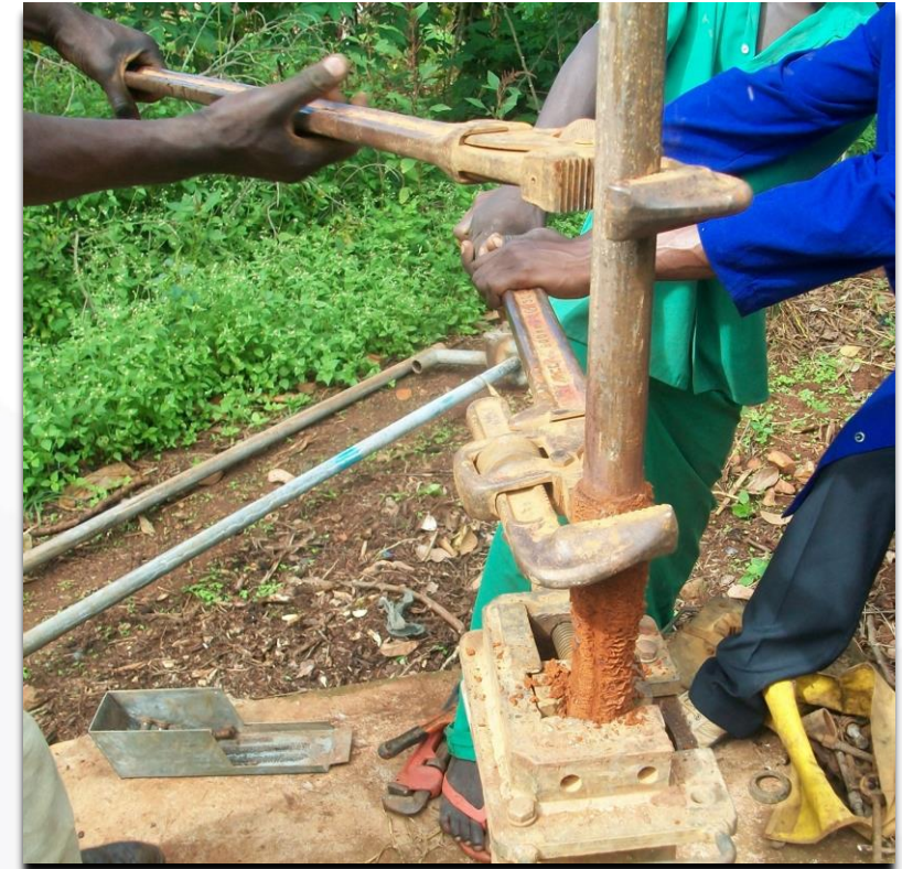
Figure: Removal of corroding riser pipe in Hoima, Uganda in 2012 (Source: Larry Bentley). Note: In 2018 the Government of Uganda issued a directive to prevent further use of Galvanised Iron riser pipes throughout the country
