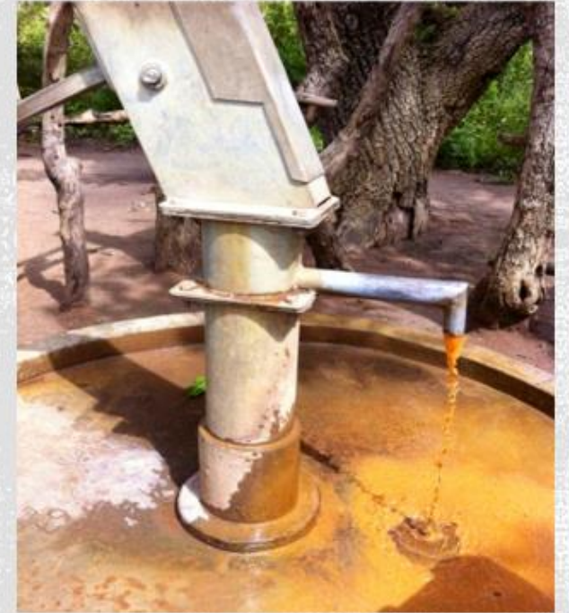
Red, iron-rich water being pumped Photo: WaterAid Uganda
