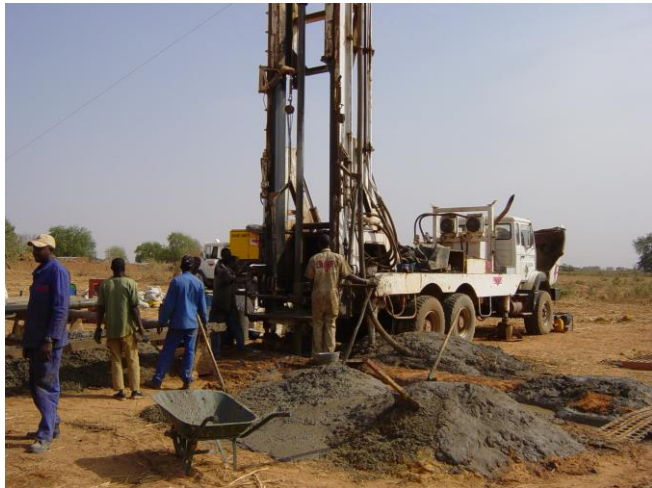
A range of mechanised rigs (Photos: Erich Bauman/Kerstin Danert)
