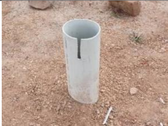
Slot in the casing to accommodate cables in the casing.
