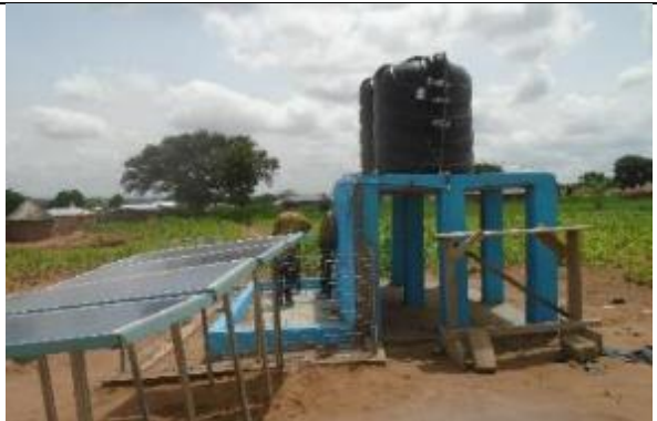
4 pumps ZL50-20N in series powered by 4 panels of 100 Watt. Water is used for communal water supply
