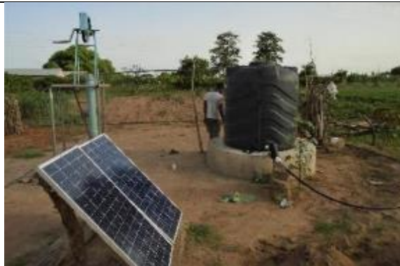
1 pump ZL 50-20N is replacing a Rope pump. It pumps into a tank and is used for drip irrigation.
