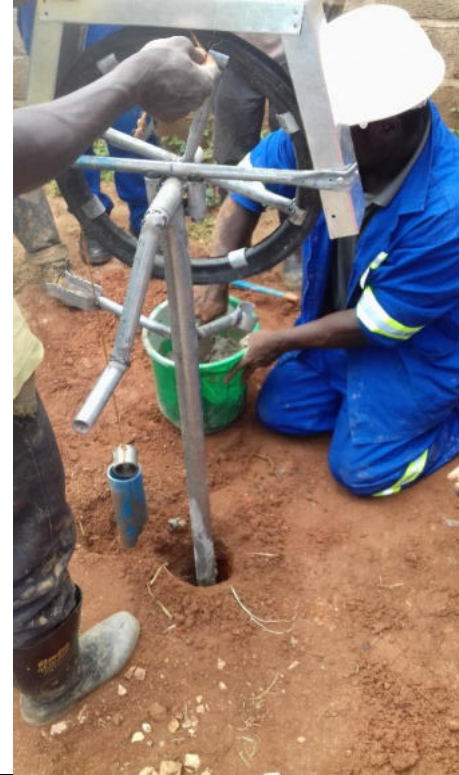
Installation of the pump on a hand drilled tube well. Distance pole to casing ca 20 cm
