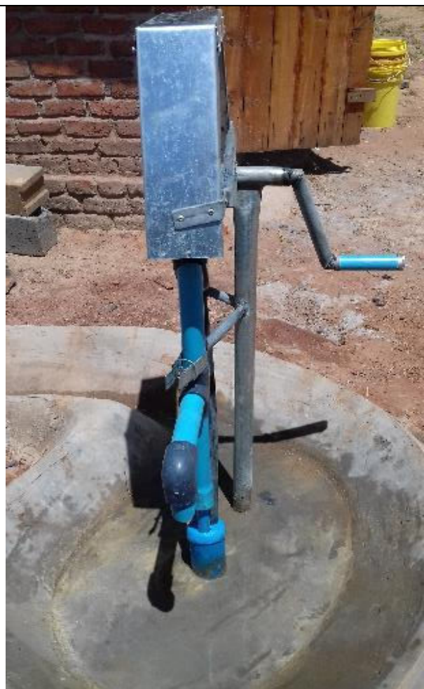
Front view Pole 0.5 m in the ground / Concrete
