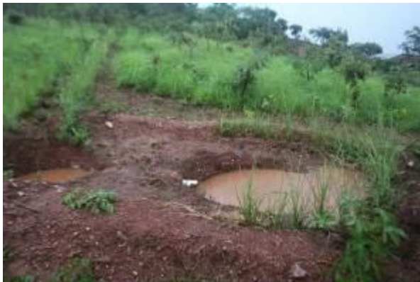
Where the recharge uses ground run off it is recommended to make 2 pits. The first pit is to let sand or clay settle so the water that flows into the second pit is relatively clean.
