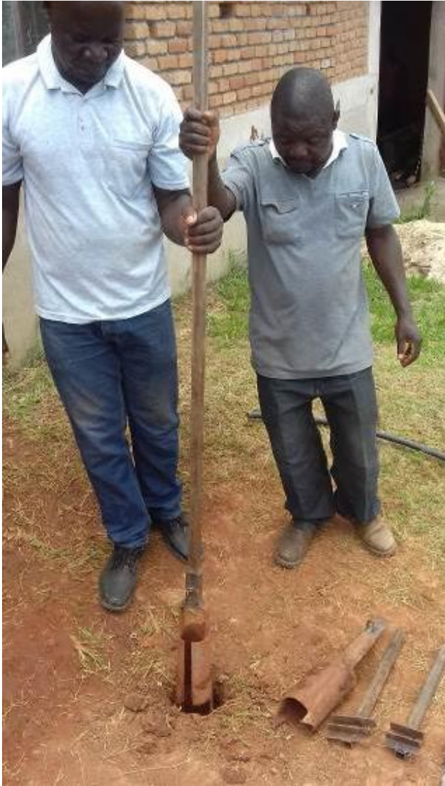
The recharge hole is made with a Core auger of 2 or 3 inch. The Auger is turned around with handles. See also manual of the Mzuzu drill.
