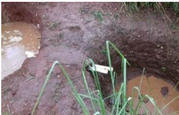
Where the recharge uses ground run off it is recommended to make 2 pits. The first pit is to let sand or clay settle so the water that flows into the second pit is relatively clean.
