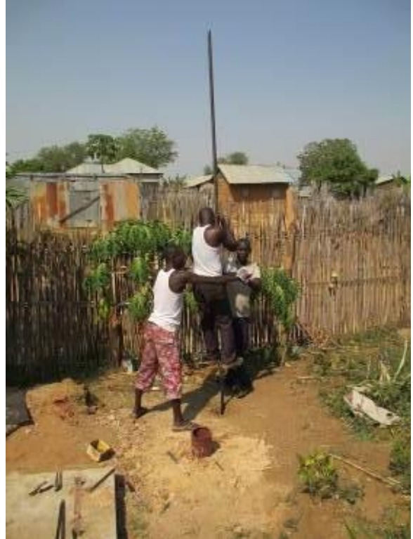
The Core auger has drill pipes of 3 meters long which can be extended with another pipe of 3m. Eventually a step can be mounted for a person to increase the weight on the auger.
