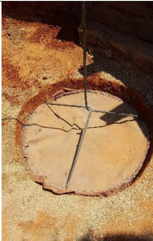
Do not completely fill the small pit Make a cloth filter that has a tight fit in the hole. The sides of the holes are a bit conical.
