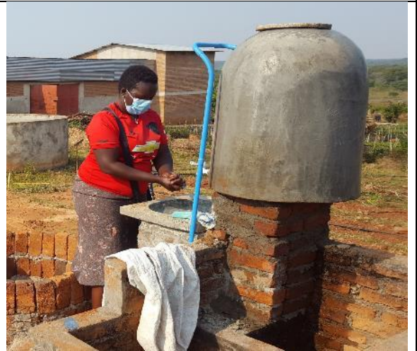
EMAS storage tanks of 80 litres and wash basin
