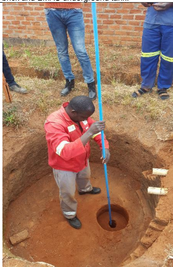
Training in the construction of a Tube recharge system.
