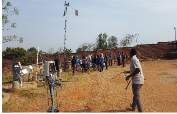
Installation of an EMAS pump in a borehole of 20 metres deep. Time needed 5 minutes
