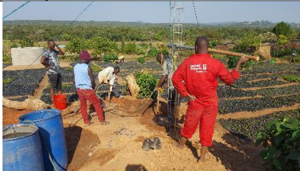
Drilling a borehole, 5 metres per hour
