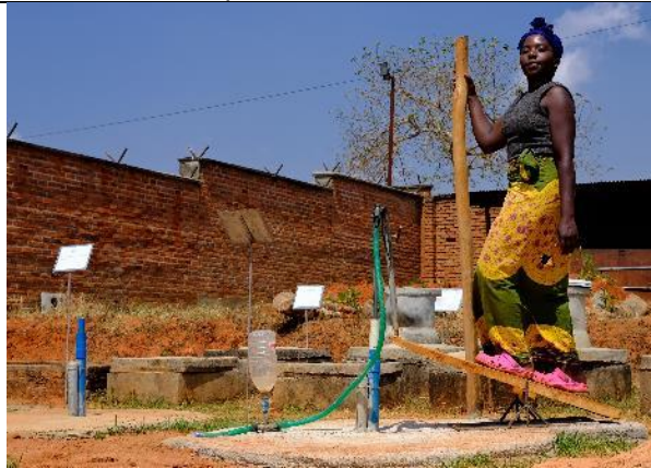
Installation of an EMAS pump in a borehole of 20 metres deep. Time needed 5 minutes
