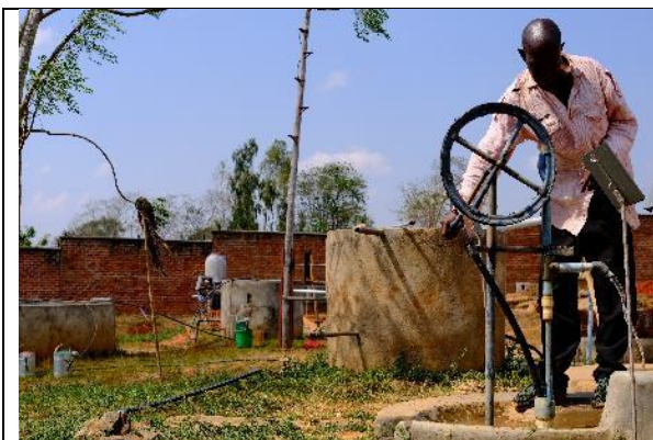
Rope pumps model 4 installed on a borehole of 2 inch ( 60 mm)
