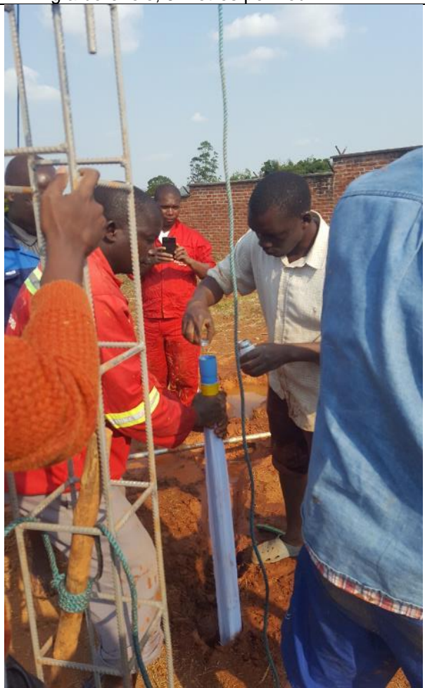
Installation of the casing pipe, 1.5 inch (40mm)
