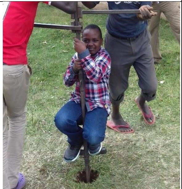
Drilling with the Mzuzu drill
