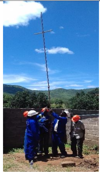
Photo 8. If the drill pipes are longer than 6 meters, take off the pipes exceeding 6 meters.
