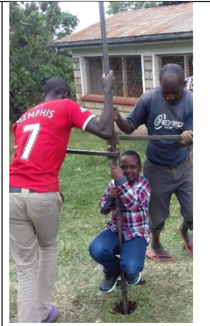
Photo 5. Use Footstep for hard ground layers. Stay close to the drill pipe
