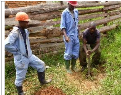
Photo 9. Using the Stone punch with the 4 steps. 1 Down, 2 Swing, 3 Lift, 4 Turn
