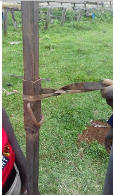
Photo 7. To remove the fast fix pin pull the rubber strip.
