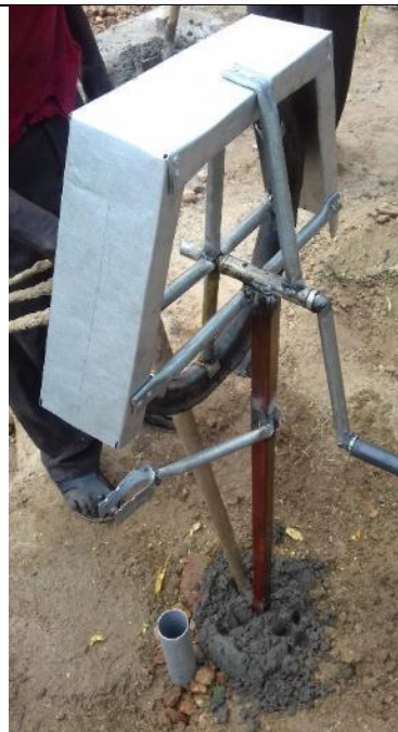
Photo 29 Putting concrete in hole and for apron
