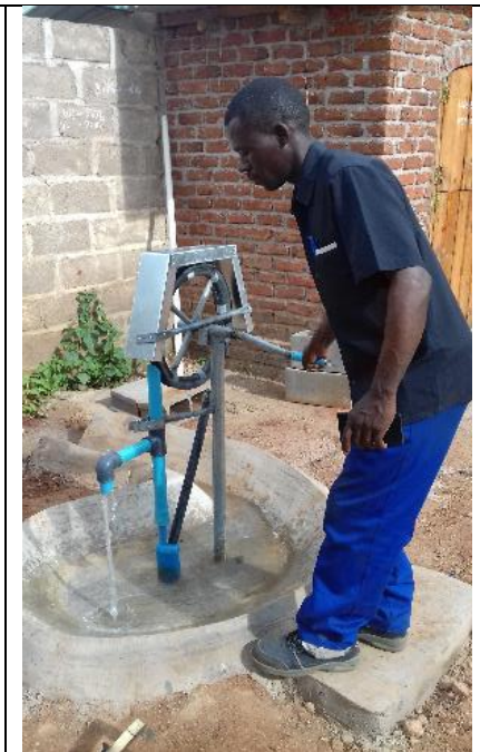
Photo 30 After pumping and swabbing the water becomes clean
