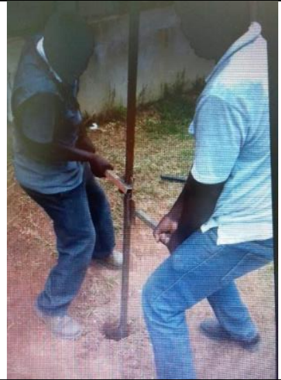
Photo 4. Lift the auger with the handles. Keep on turning to the right while lifting
