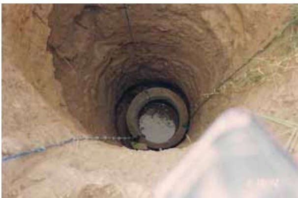
Top photo: A well completely lined with cement rings.
