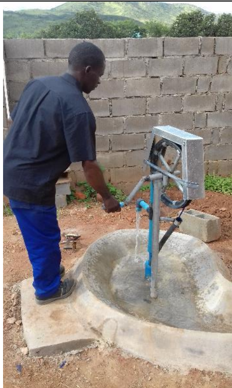
Rope pump model 4 with a removable wheel cover. Pole of GI pipe 1¼".
