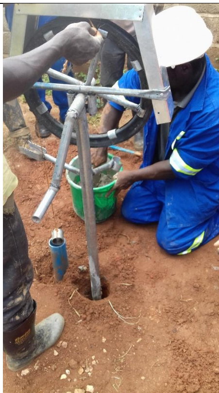
Installation of the pump on a hand drilled tube well. Distance pole to casing ca 20 cm
