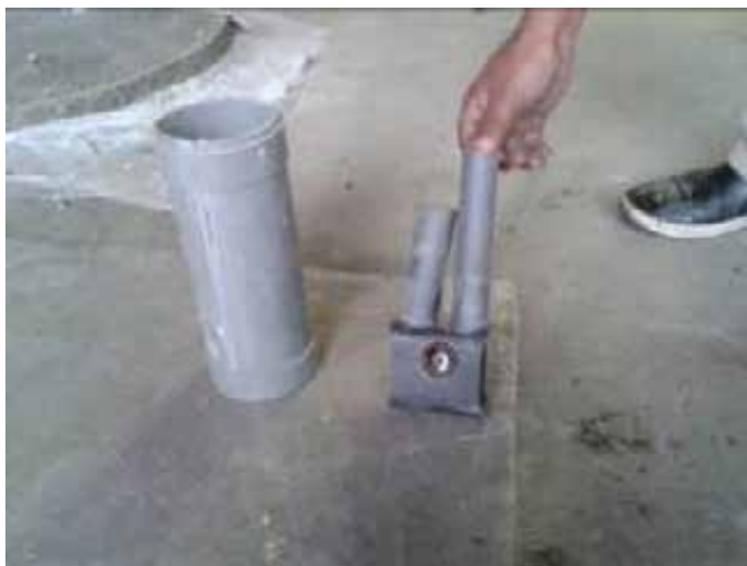
Making cement guideblock
