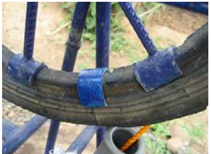
Here clamps are installed but length is not good
