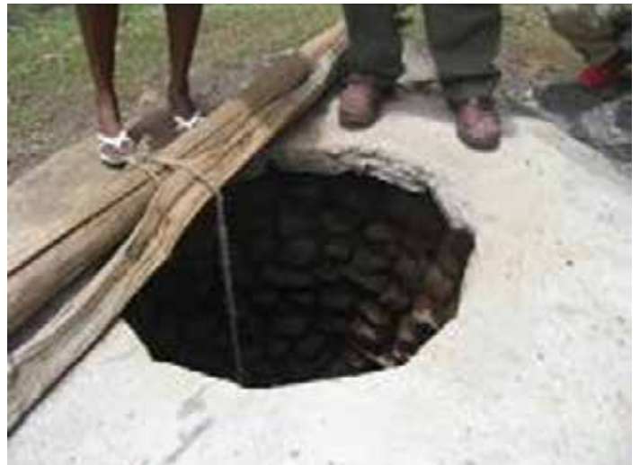
Well reducer ring made of tapered blocks
