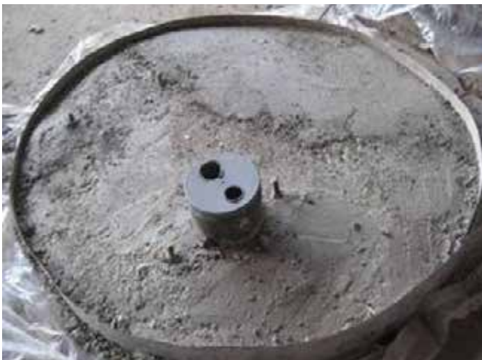
Finished well slab
