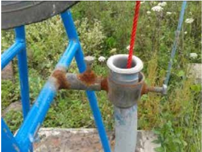
Corrosion of bolts, trumpet on return pipe poor quality
