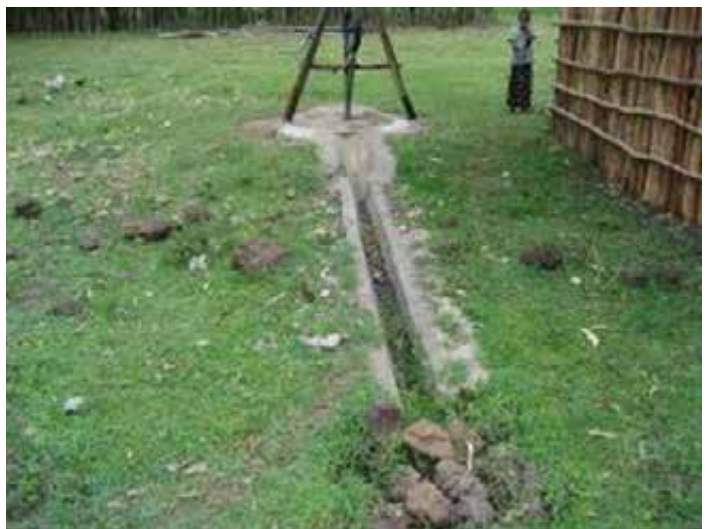
Good example of Soakpit, all water goes to the pit. The pit is filled with stones so no water is visible so not drinking of cows, no mosquitos etc.
