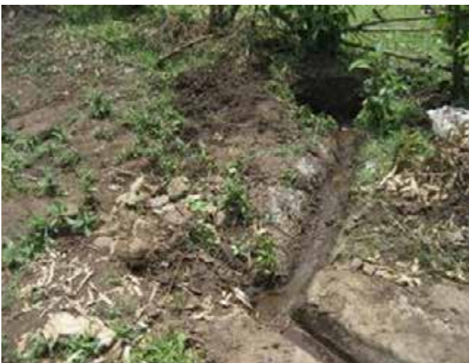
Bad example of Soakpit, The pit with stones was blocked and a new hole for cattle was made. This results in contaminated water.
