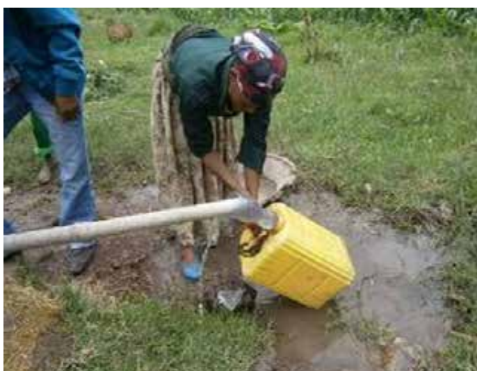
Large diameter outlet pipe so pipe does not fit into the jerrycans. Suggestion to reduce diameter outlet pipe to 1 1/4"
