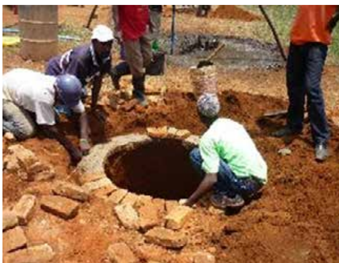
Making well ring reducer with bricks
