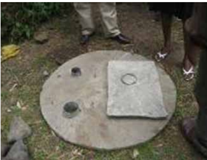
Well cover with Manhole. Water can leak back in well since there is no rim around the hole.
