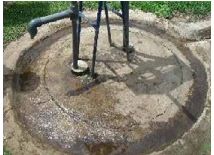
Here the well slab is not sealed well on the well rim.
