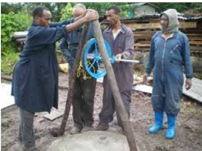
Installing pole model pump
