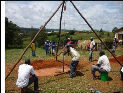
SHIPO drill. A manual drilling option combining percussion and sludging. Depths to 50 metres. Ca 800 wells drilled
