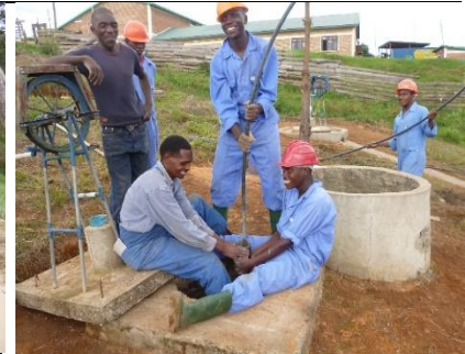
Well Pipe.. Hand dug wells that dry up can be made deeper with a Well pipe system which uses a Tube bailer inside a 4 inch PVC casing
