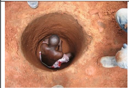
Small diameter wells. Digging a well of 0.7Meter diameter is 50% less soil removal than a well with a diameter of 1 meter.
