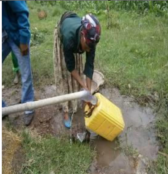
Large diameter outlet pipe so pipe does not fit into the jerrycans. Suggestion to reduce diameter outlet pipe to 1 1/4"
