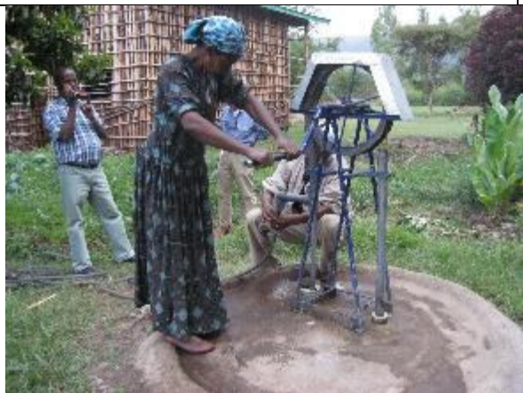
Here a hose is connected to the outlet to transport water to the garden on the other side of the house
