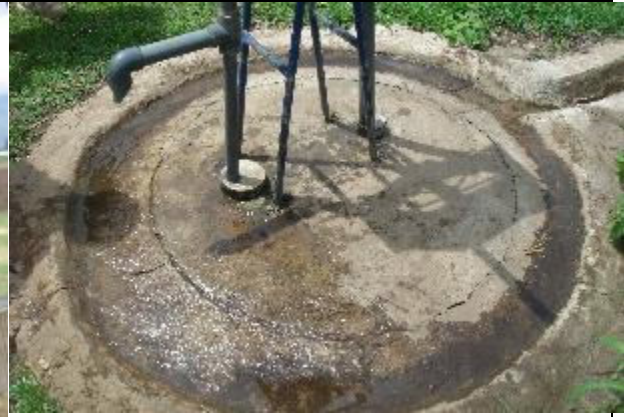
Here the well cover is not sealed on the well rim.
