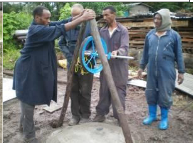
Installing pole model pump
