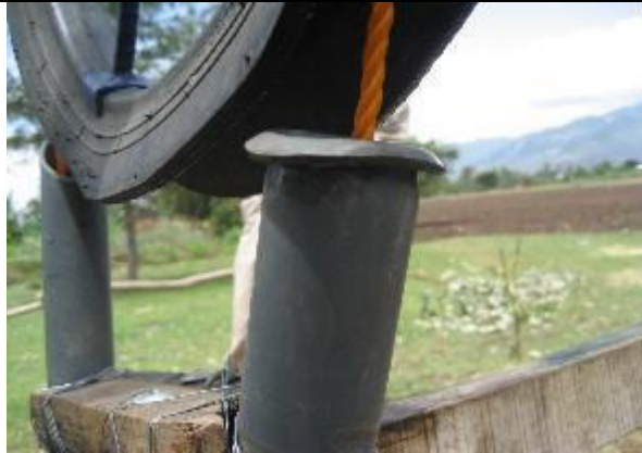
The inlet of the return pipe is not good. It requires a nice smooth entrance, a so called trumpet which can be made with a trumpet tool.
