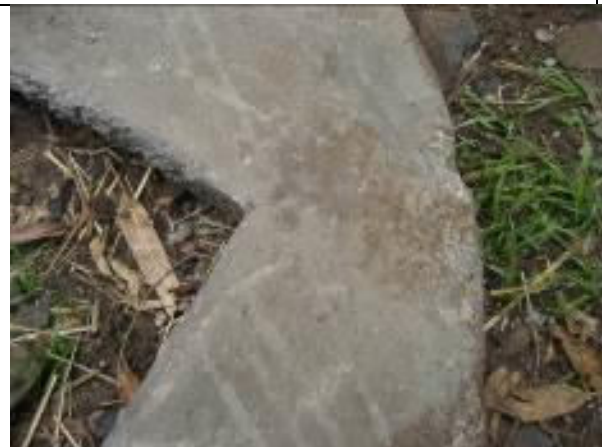
The manhole makes the well cover weak. Like in this case there is a crack cracked in the corner so another source for leaking water in the well.
