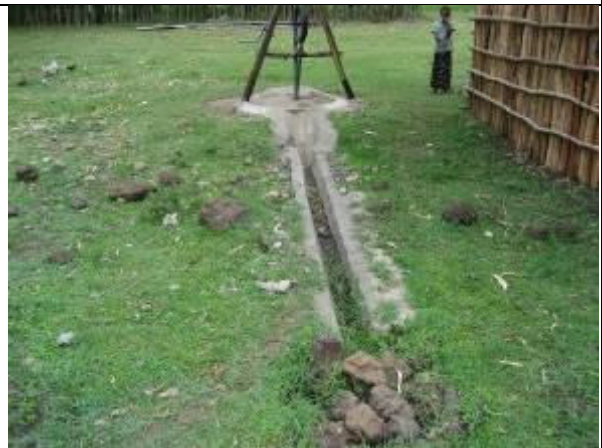
Good example of a Soakpit, all water goes to the pit. The pit is filled with stones so no water is visible so not drinking of cows, no mosquitos etc.
