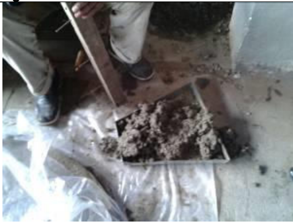
Using a mould to producing concrete blocks for a well ring
