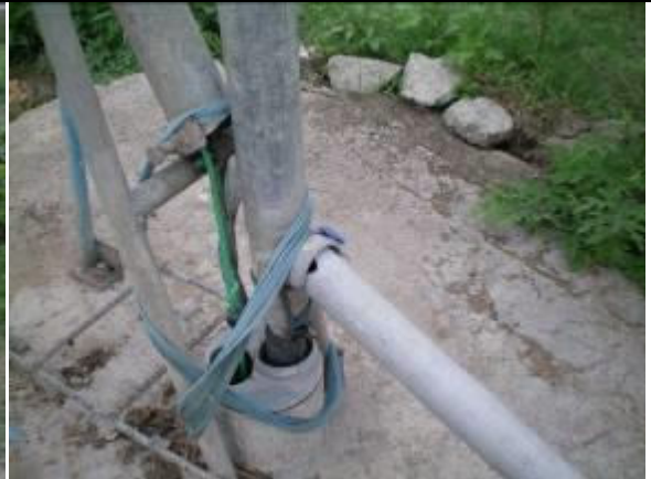
Return pipe not sealed, PVC parts broken, Pipe end cap is cut and has large holes so water leaks back in well.
