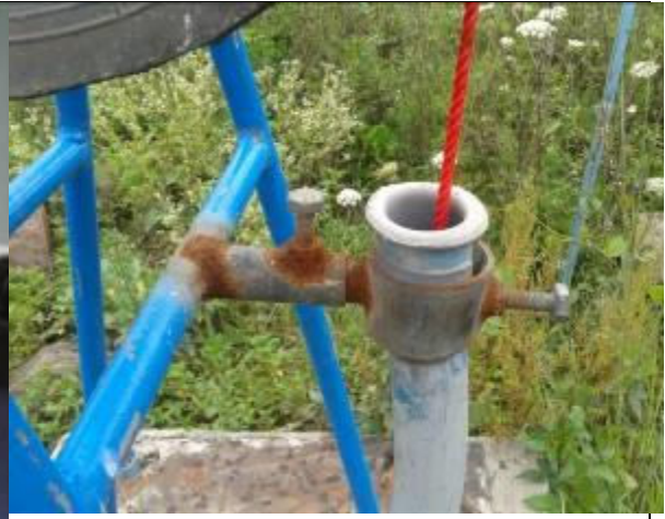
Corrosion of bolts, trumpet on return pipe poor quality
