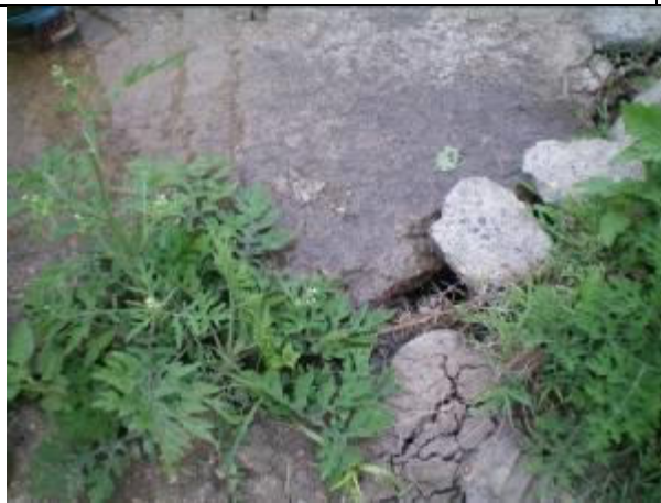
Lack of apron so water leaking back in well
