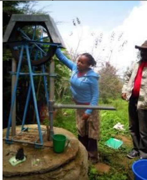
Pump high since it is mounted on a parapet. In this case short base model should have been used or a platform should be installed.
