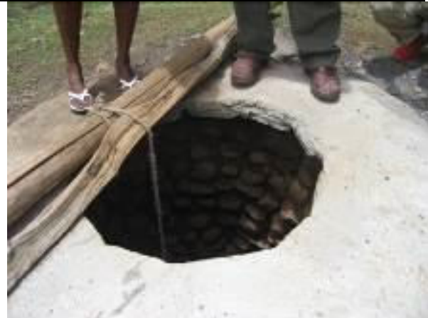
Well reducer ring made of tapered blocks
