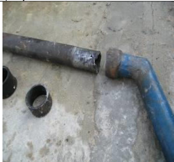
Lack of oiling resulting in broken handles
