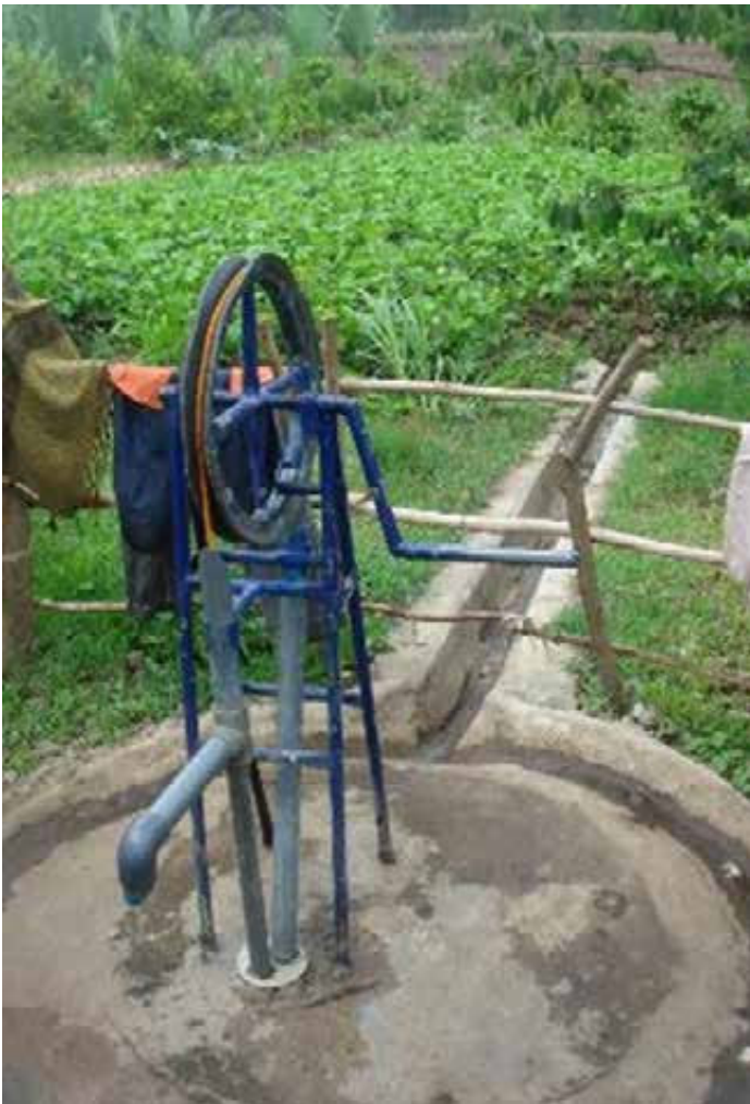
Rope pump Model 2, with a return pipe, without wheel cover. Used for irrigation of a garden.
