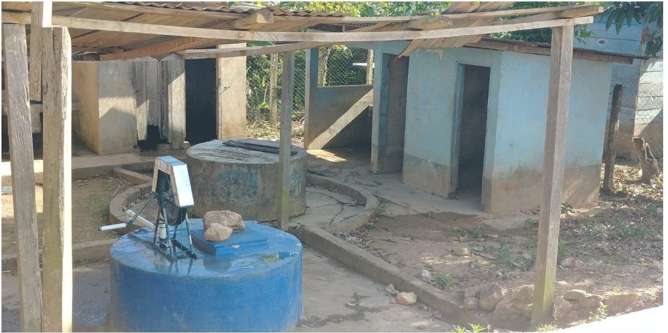
Photo 10: Functioning rope pump on community waterpoint, hand dug well (Las Brenas, Municipio Rosita, RACCN)
