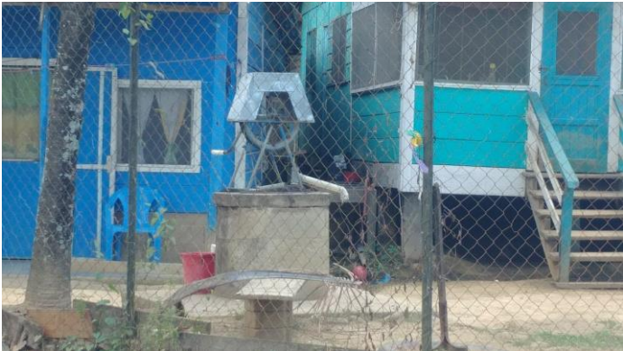
Photo 14: Functioning rope pumps on family hand dug wells in urban area (Rosita, RACCN).
