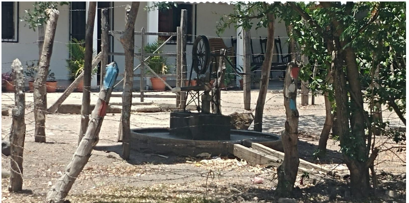
Photo 13: Functioning rope pump on communal water point, borehole well (Municipality of Boaco)
