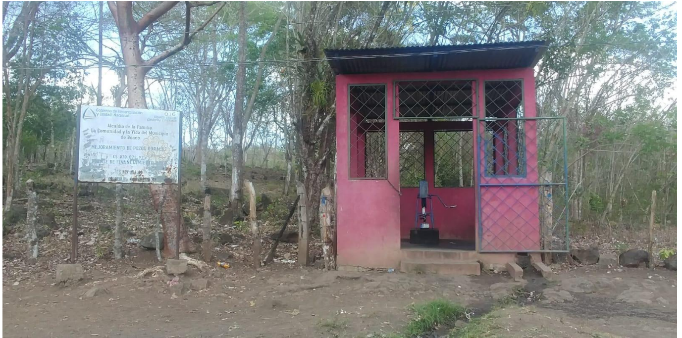
Photo 12: Functioning rope pump on communal waterpoint (borehole well) rehabilitated in 2016 (Municipality of Boaco).
