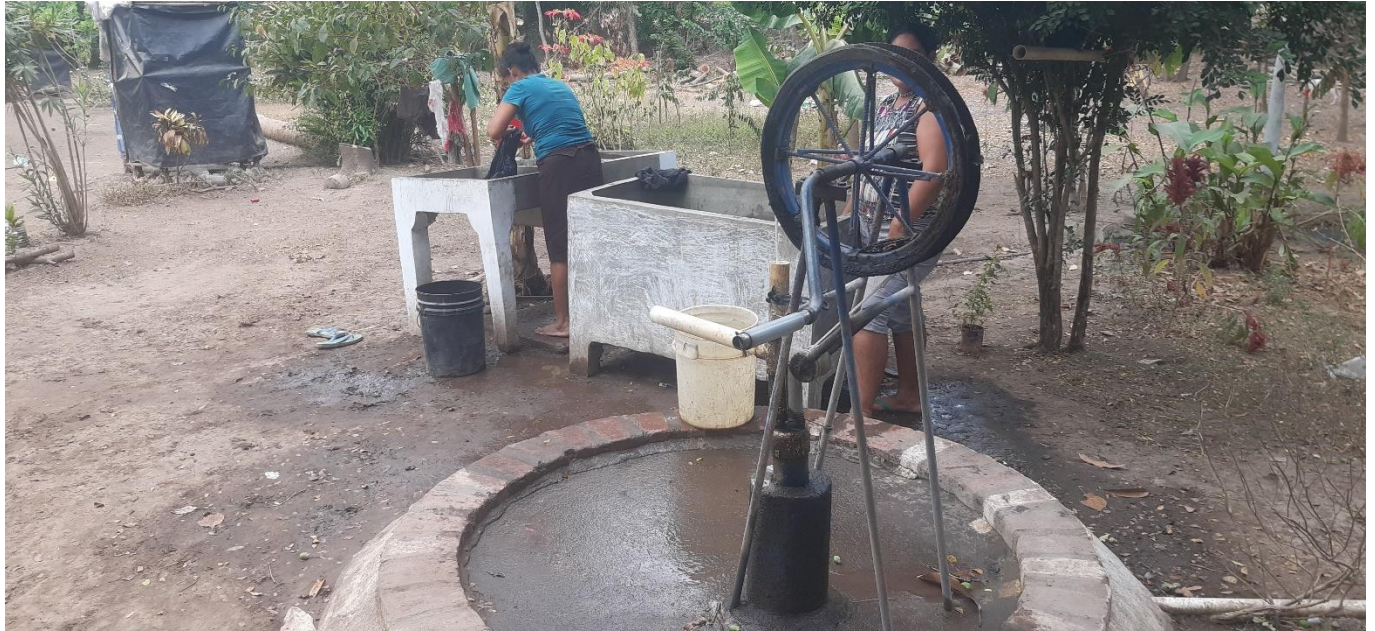
Photo 6: A still functioning original rope pump on family well (shared by two households) used for human consumption, washing, bathing and irrigation of patio garden, Matapalo village.
