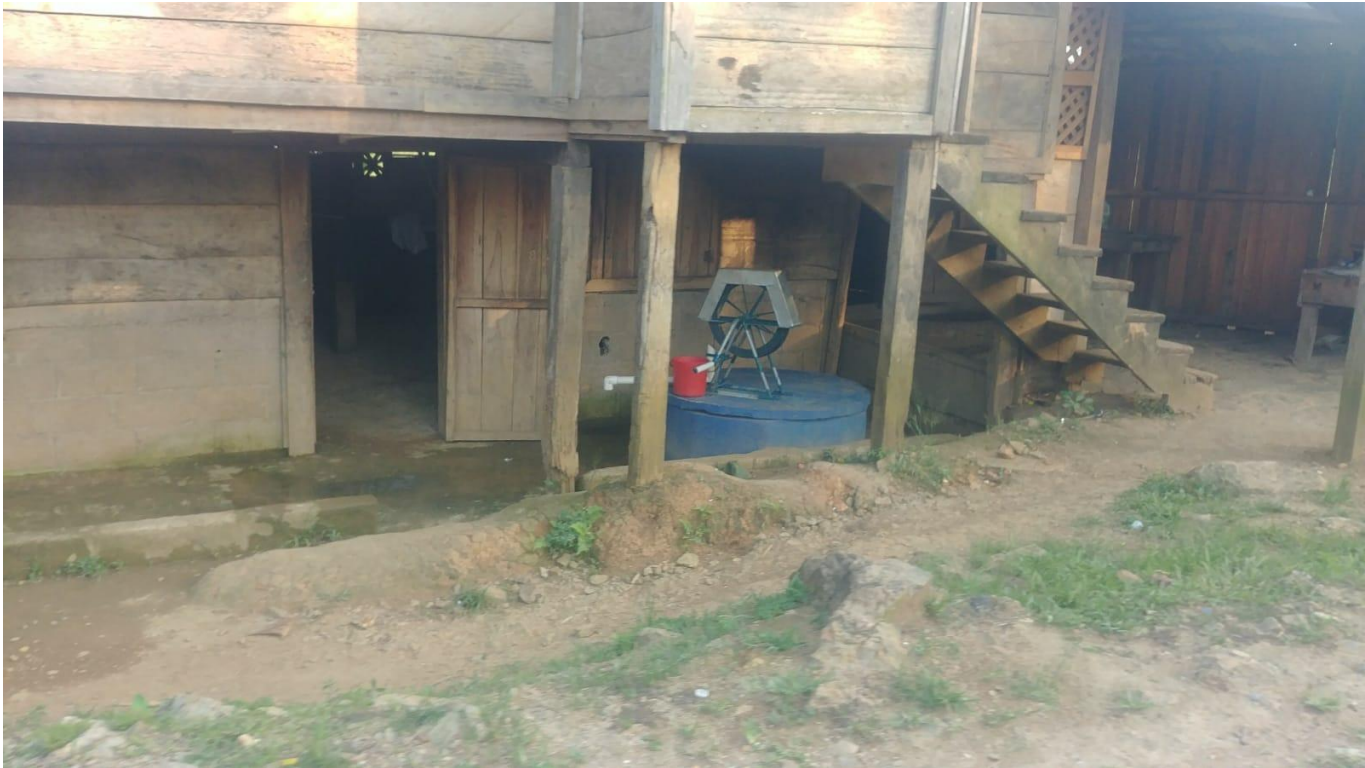
Photo 15: Functioning rope pumps on family wells, hand dug (Municipality of Rosita, RACCN).
