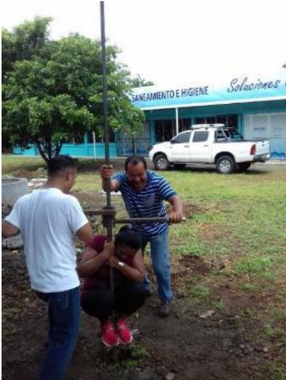
Drilling with a core auger. 1 person on the Foot step to increase the weight.
