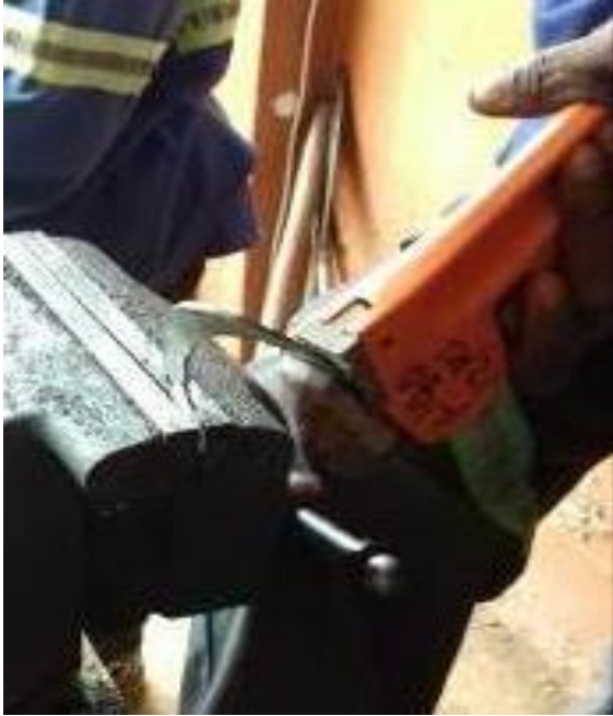
Bend the plates in a vice until opening is 40 mm or more. Weld the plates on a ½" GI pipe
