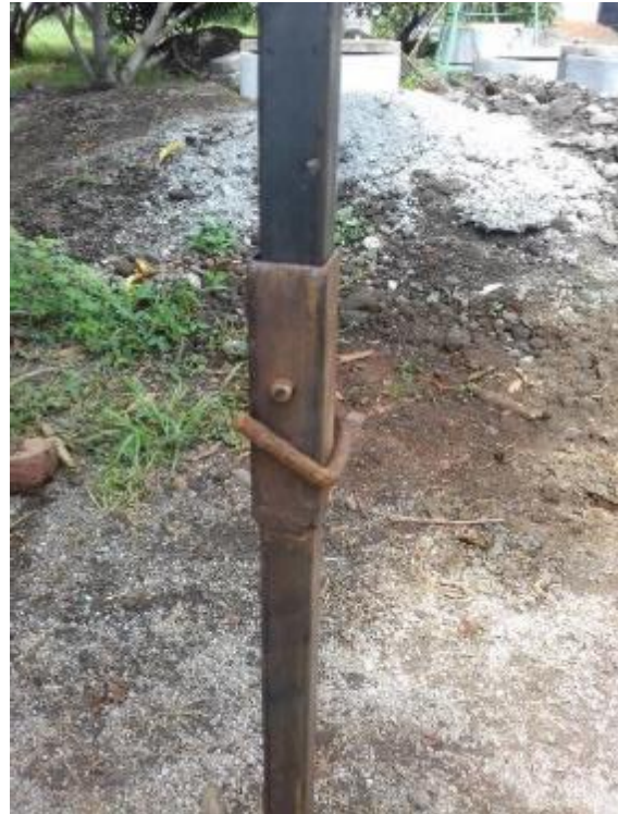
The fast fix pin to connect 2 drill pipes
