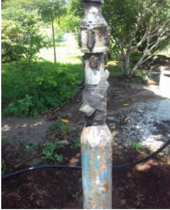
Use rubber strip to make sure it is closed completely
