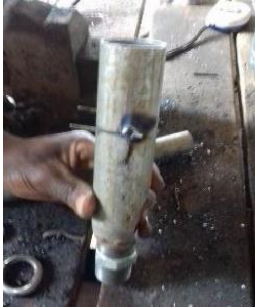
To fix the valve inside the 2 inch pipe, make 2 cuts and weld pieces of welding rod.
