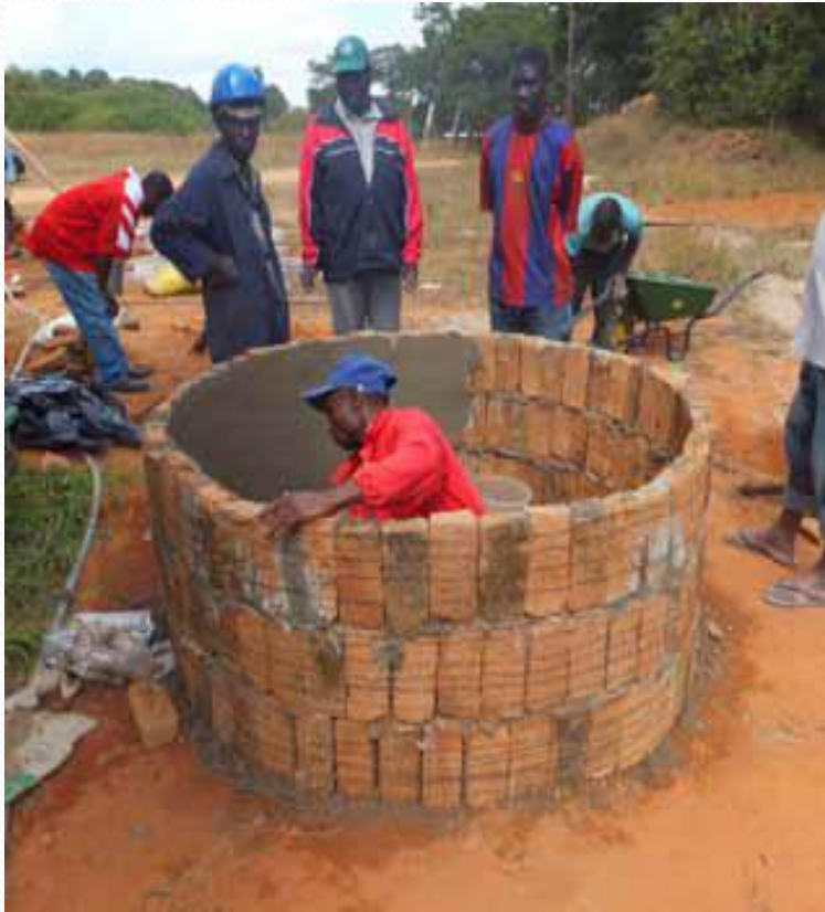
Wire-brick cement tank,
