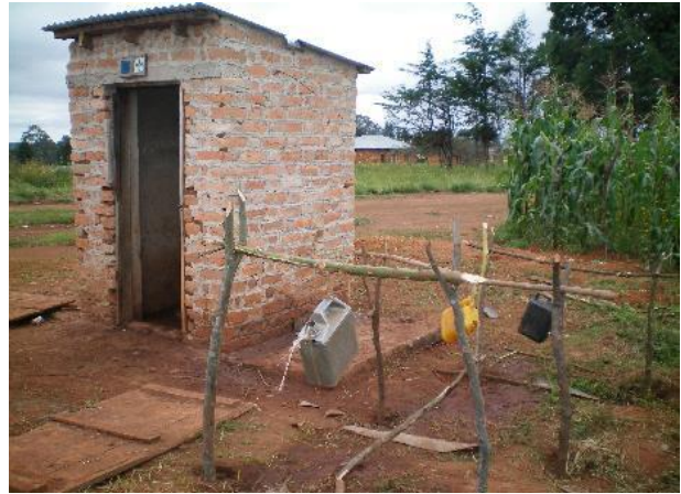
If possible install Tippy taps near latrines
