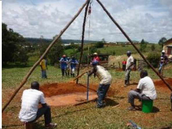
Drilling a tube well of 30 meters deep with the SHIPO drill method
