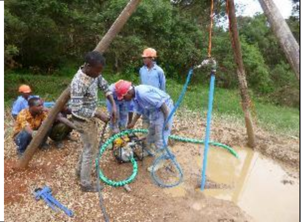
The SHIPO drill combined with jetting
